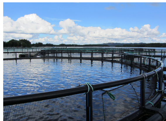
Figure 3. Basic diagrams showing cage farms. The structure consists of an anchoring arrangement, a floating structure and a net cage.
